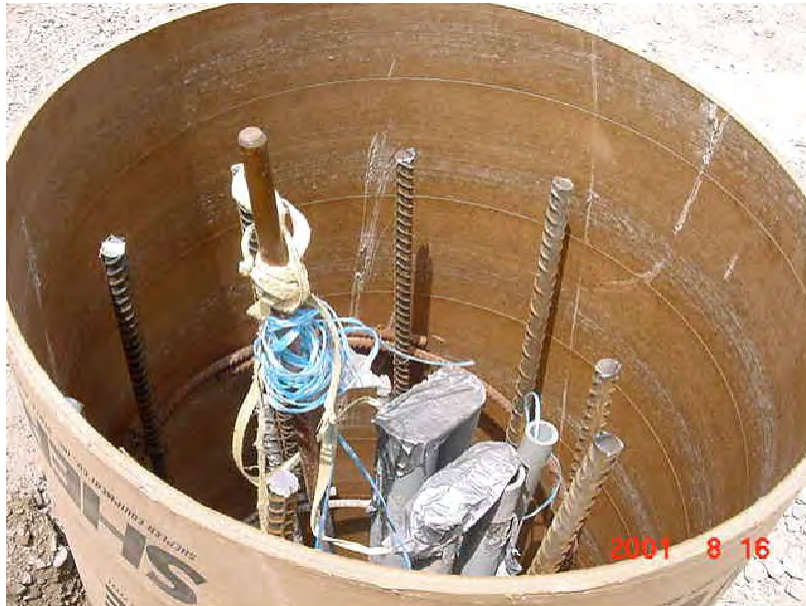
FIGURE 9.9.4 REBAR, ELECTRICAL CONDUIT
